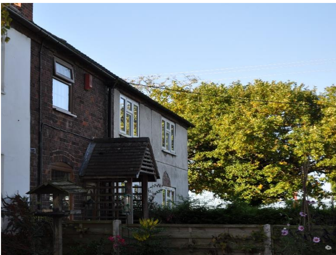
View of the north facing front façades of Orchard Cottage (to the left) and Boroughfields Farm Cottage (to the right).
