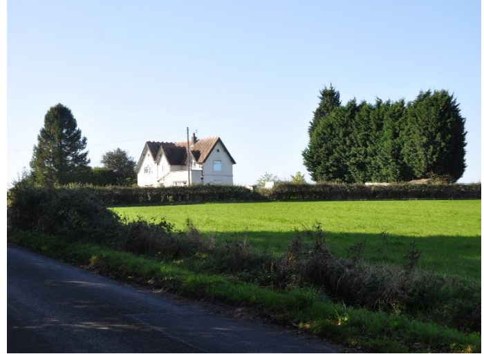
View of property showing eastern façade (to the left) and western façade (to the right).
