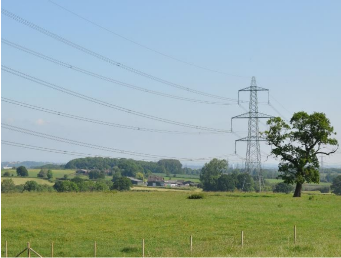
View of the south facing façade seen beyond light industrial units, taken from the western edge of field O5.
